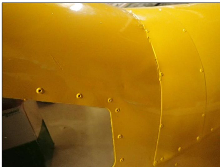
Photo No. 4 and Photo No. 5 : Wrinkling of aircraft skin
